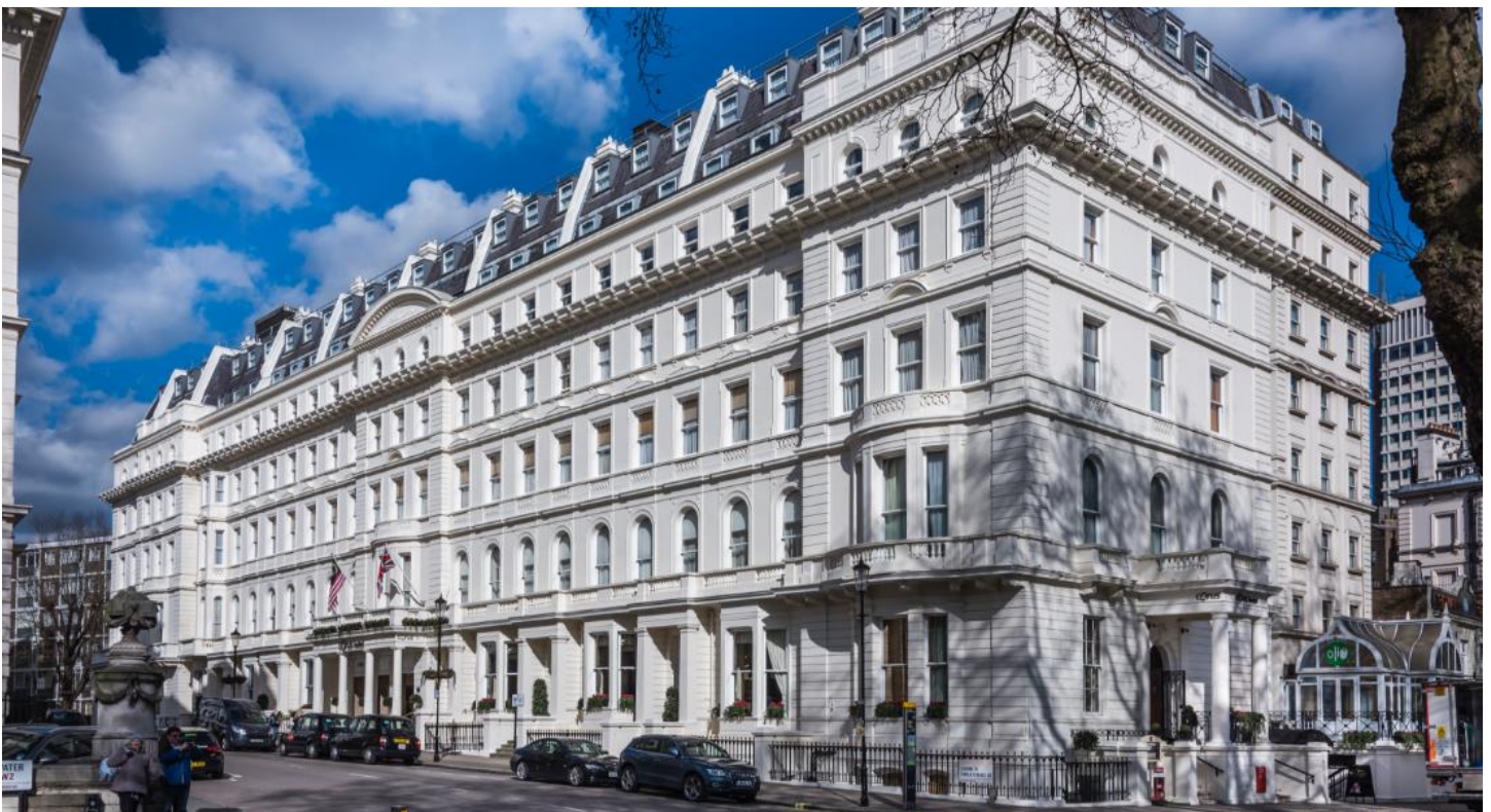
Exterior of the Corus Hotel | Hyde Park.
